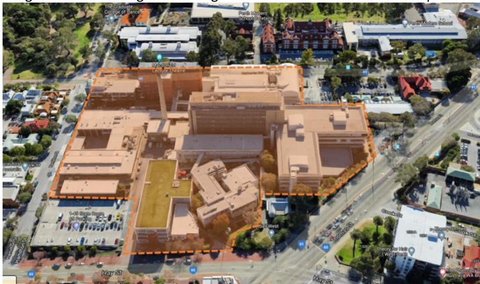
Figure 2. PMH Demolition Area
