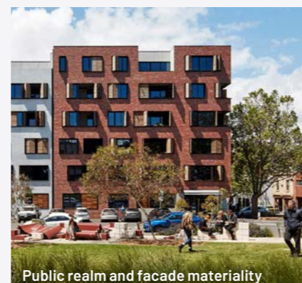
Public realm and facade materiality
